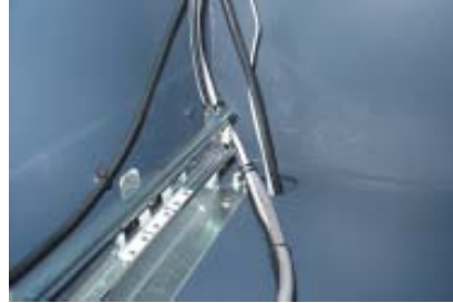
Figure 1. Power/phone cable routing.
