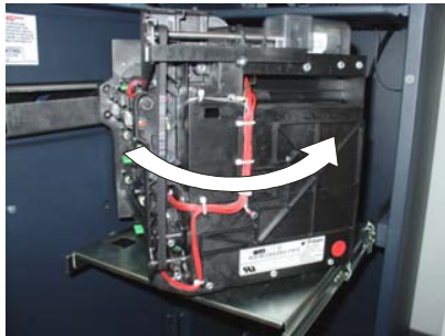
Rotate mechanism to operate position (counterclockwise).
